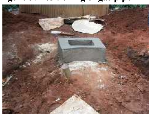
Figure 5: Digester covered with the soil
