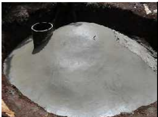
Figure 2: Surface finishing
